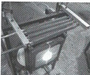
Fig. 9 STARworks Glass Lab's glory hole waste heat exchanger heats 40 gallons of water from 78°F to 122°F in one hour
